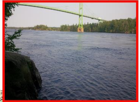
View of 1000 Islands Bridge from Campsite 106
